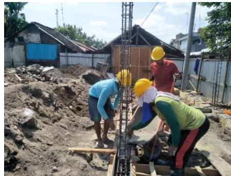
Gambar 4.7 Proses Pengecoran Sloof
