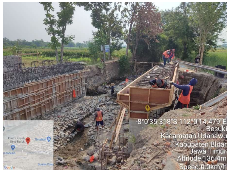
Gambar 6.8 Pekerjaan Ground Shield
