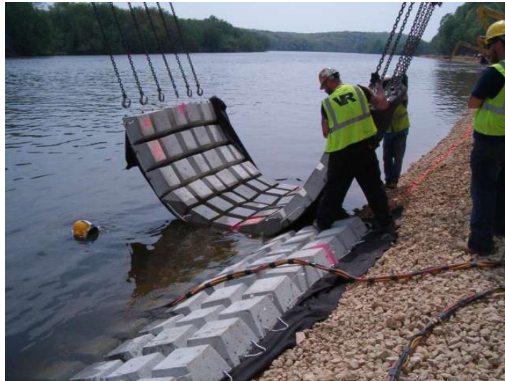
Gambar 2.17 Penerapan Concrete Mattress di Dasar Sungai
