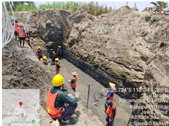
Gambar 6.4 Galian Dasar Talud
