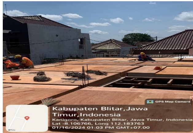
Gambar 3.2 Triplek / Plywood
