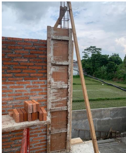
Gambar 3.7 Bekisting Kolom
