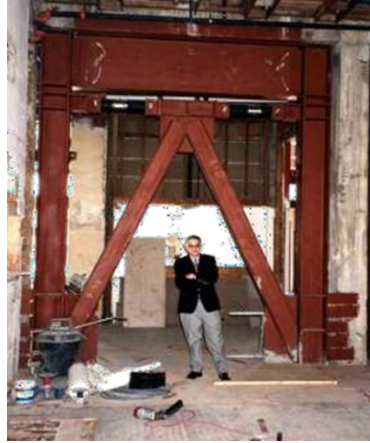
Gambar 2. 5 Pemasangan Damper The Hotel Woodland, Woodland, California.
