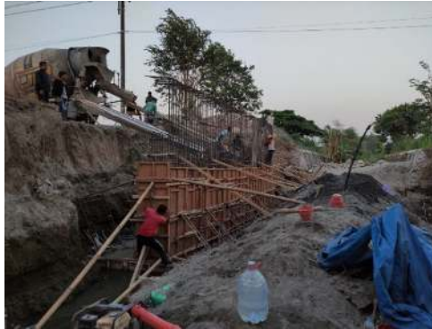
Gambar 4.23 Pengecoran Abutment A
