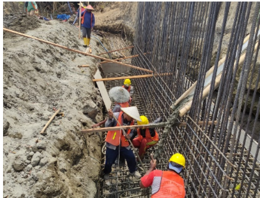
Gambar 4.22 Pengecoran Pondasi Abutment A
