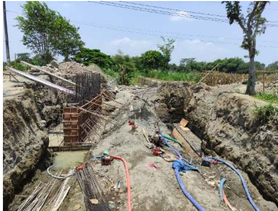
Gambar 4.19 Pekerjaan bekisting abutment A
