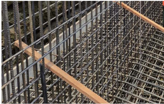
Gambar 4.4 Besi tulangan ulir (sirip) diameter 16 mm
