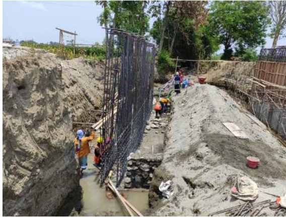
Gambar 4.18 Pembesian Abutment B
