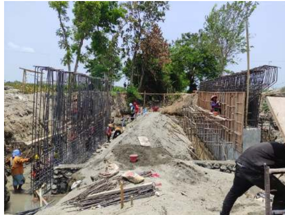
Gambar 4.20 Pemasangan Beksiting Abutment A
