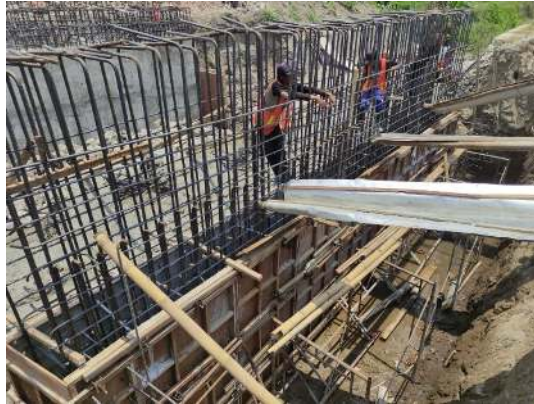
Gambar 4.26 Pengecoran Abutment B
