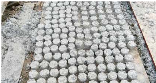
Gambar 4.6 Decking beton
