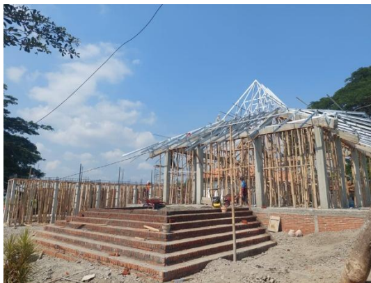
Gambar 4.30 Rangka Galvalume by Applicator (Sumber : Data Lapangan, 2023)
