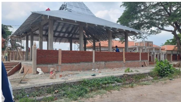
Gambar 4.31 Atap dilapisi Aluminium Foil Bubble (Sumber : Data Lapangan, 2023)
