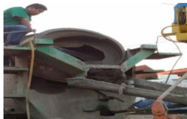
Gambar 4.10 Concrete Mixer Truck (Sumber : Kerja Praktek 2022)
